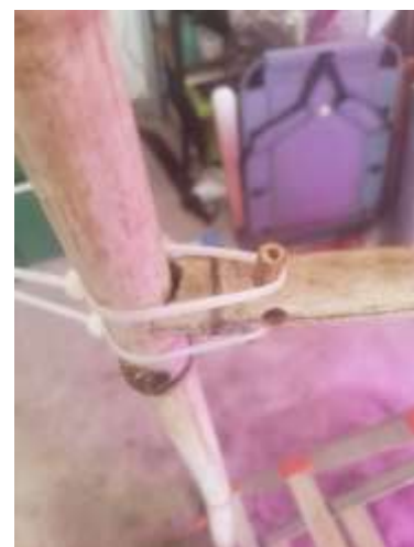
Figure 7 – Bamboo dowel pin and twine (zip-tie)
